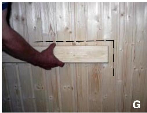
**F.** Notice that 2 bench supports have already been attached to the interior of panel 6. You will now need to attach both an upper and lower bench support to panel 5.
