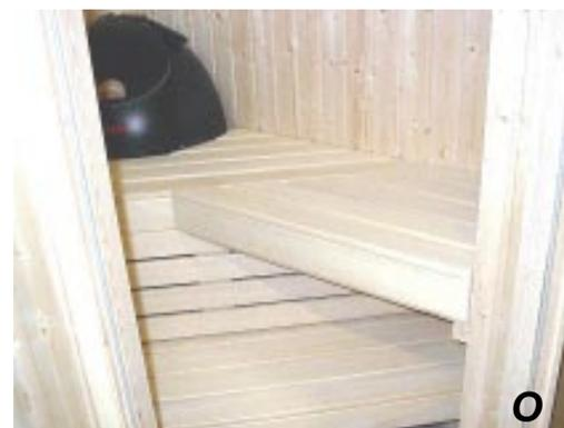
**M.** Fasten your upper bench skirt to the walls using 2 screws on each side. **NOTE:** This bench skirt is not fastened to the upper bench frame like standard bench skirts.
