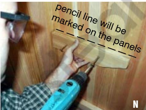
**NOTE:** Two 3/8" holes have been drilled through the frame of the upper L-bench. With the top of the benches aligned, use a 3/8" drill bit and drill through the 2 provided holes and through the face of the main upper bench. Bolt the two benches together using the 5-1/2" carriage bolts provided (photo O). Custom designed rooms may have a different bench configuration.
