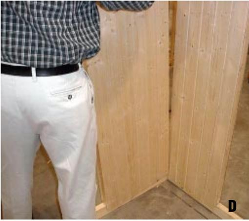
**5** Start your wall panel assembly in a corner. **NOTE:** It is not always necessary to install your panels in sequence according to their numbers. Two wall panels make up each corner. Slide one panel along the base frame until its 2x2 framework is flush with the outside of the base frame (diagram A, panel 3).
