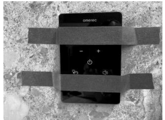
**Step 5:** After silicone has cured, remove tape and installation is complete. Control is now ready to use.
