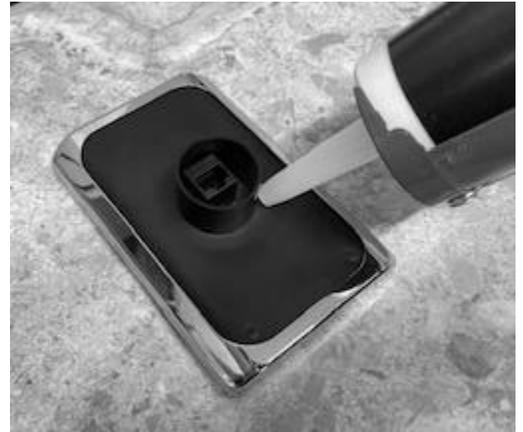
**Step 4:** Connect cable to the control. Ensure that there is a firm connection. Insert the control's tube into the mounting hole and firmly press the control against the wall. Level the control and tape it securely in place [painters tape generally works well] and leave in place until the silicone has cured completely.
