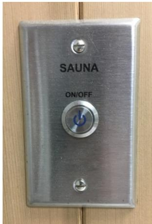
When the momentary switch is activated, the power icon will illuminate in blue and activate the sauna session that has been programmed on the SL2-C. Pressing the switch when it is illuminated will remove power to the sauna heater and end the bathing session.
